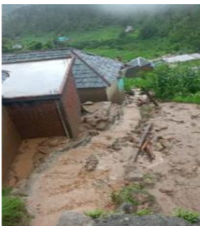
Speda Village (LHS Photo), Boh Valley Cloudburst (21 Jul 2026)
