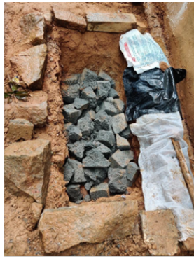
Sock pits constructed Suchitwa Mission with help of locals
