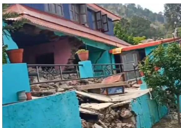
Collapsed Houses Source: Media
