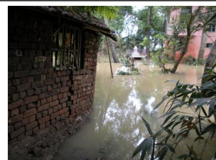
Photo showing structural damage to houses in East Chilka village
