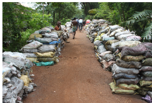
Mud sack is ready for repairing the embankment
