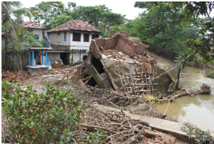
Damaged concrete house in Purba Chilka
