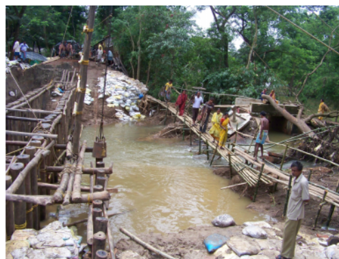
The Embankment is being repaired
