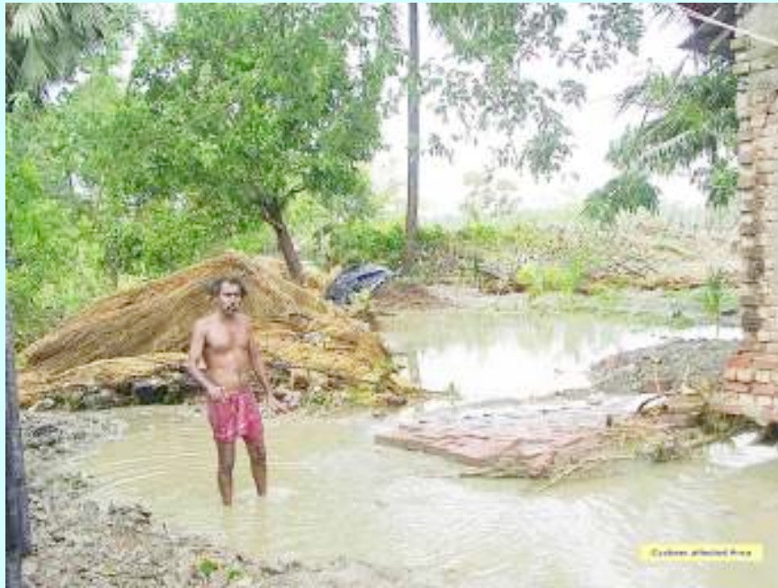
Flooded village with collapsed mud walled house on left and partially damaged brick house on right
