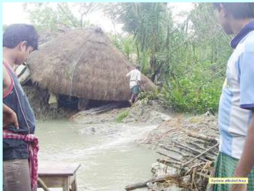
Villagers salvaging belongings from a collapsed hut of a villager. Note the hay roof collapsed on the ground as the walls are of mud
