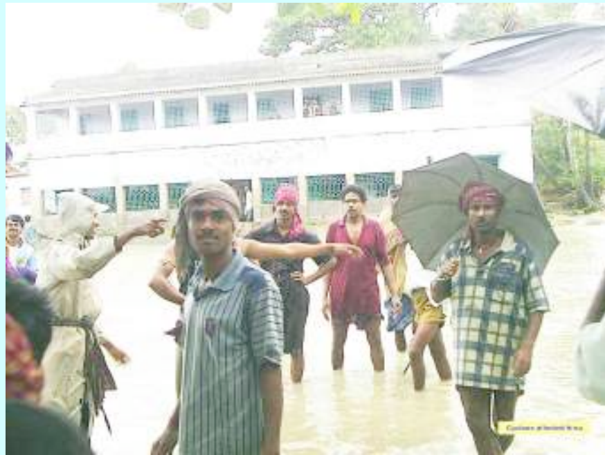
Shows flooded school playground and displaced people sheltered on the first floor
